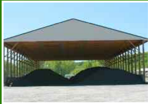
Rap Storage Facility
